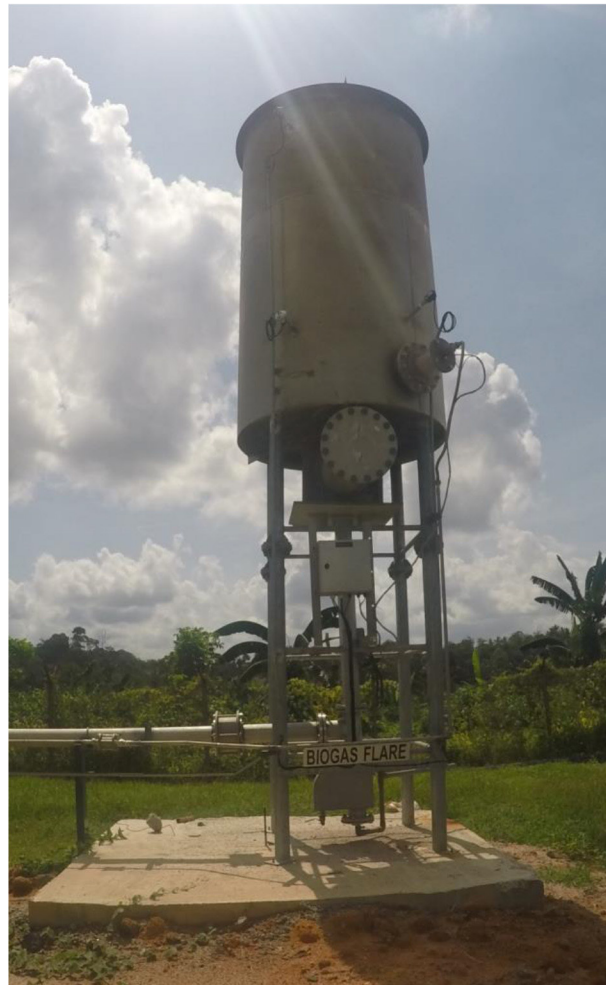
Figure 16: Open Flare (Source: FGV)
