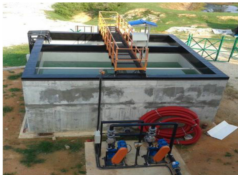
Figure 6: Above ground mixing pit (Source: FGV)
