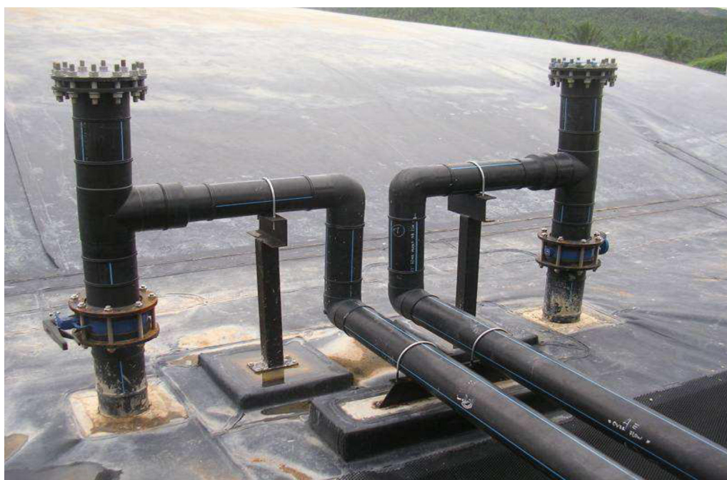
Figure 18: Digester pipeline (Source: FGV)
