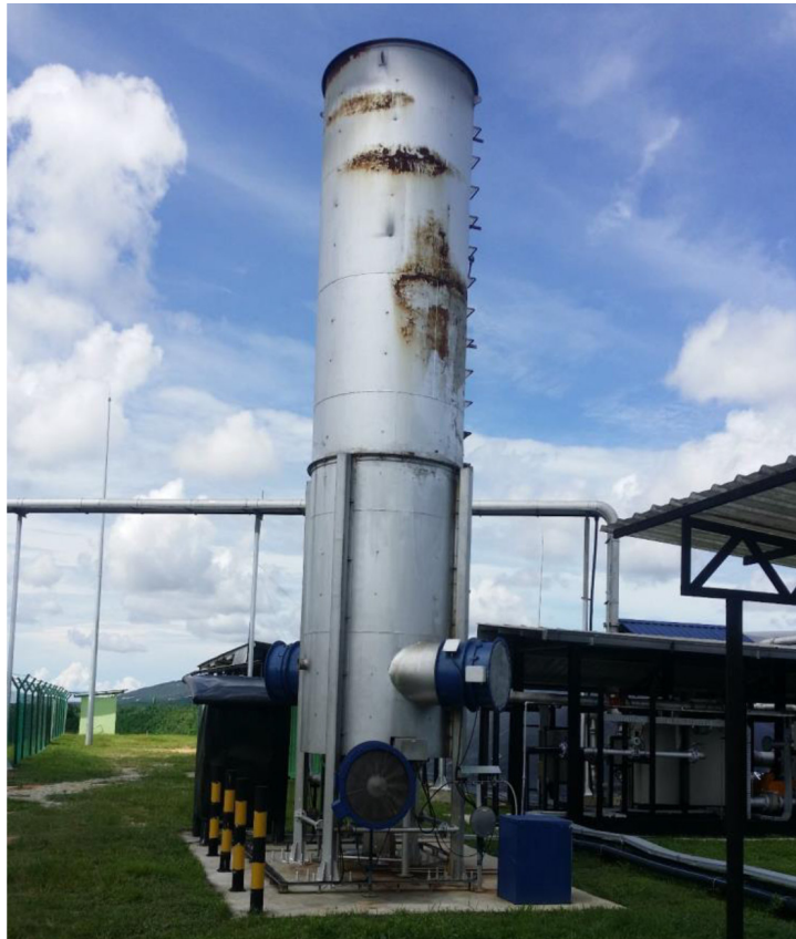
Figure 17: Enclosed Flare (Source: FGV)
