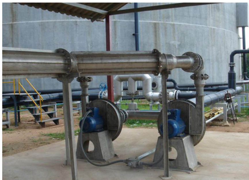
Figure 13: Blower piping system (Source: BKE Combustion Control)
