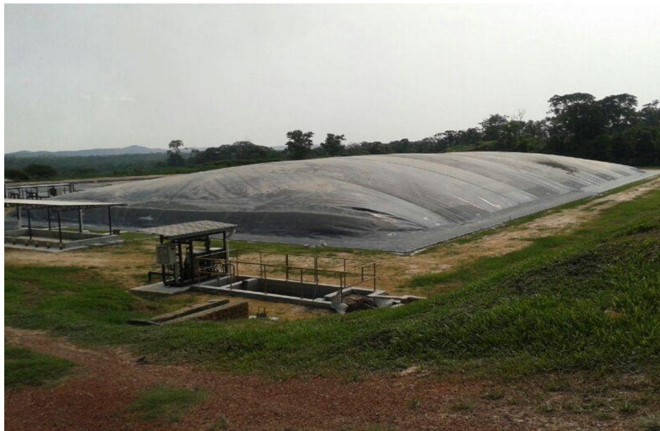
Figure 11: CA digester pond (Source: FGV)
