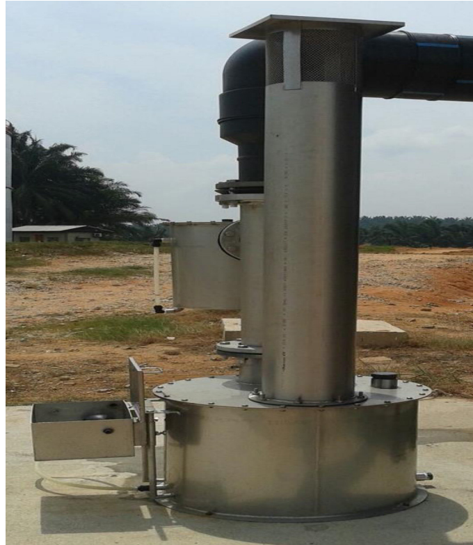
Figure 29: Pressure Relief Valve (Source: FGV)
