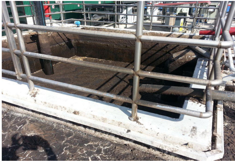
Figure 7: Under Ground Mixing Pit (Source: FGV)
